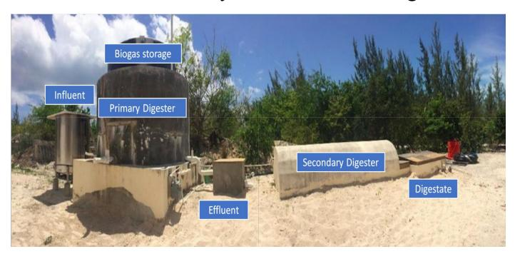
Figure 5: Anaerobic digester at Center for Sustainable Development
