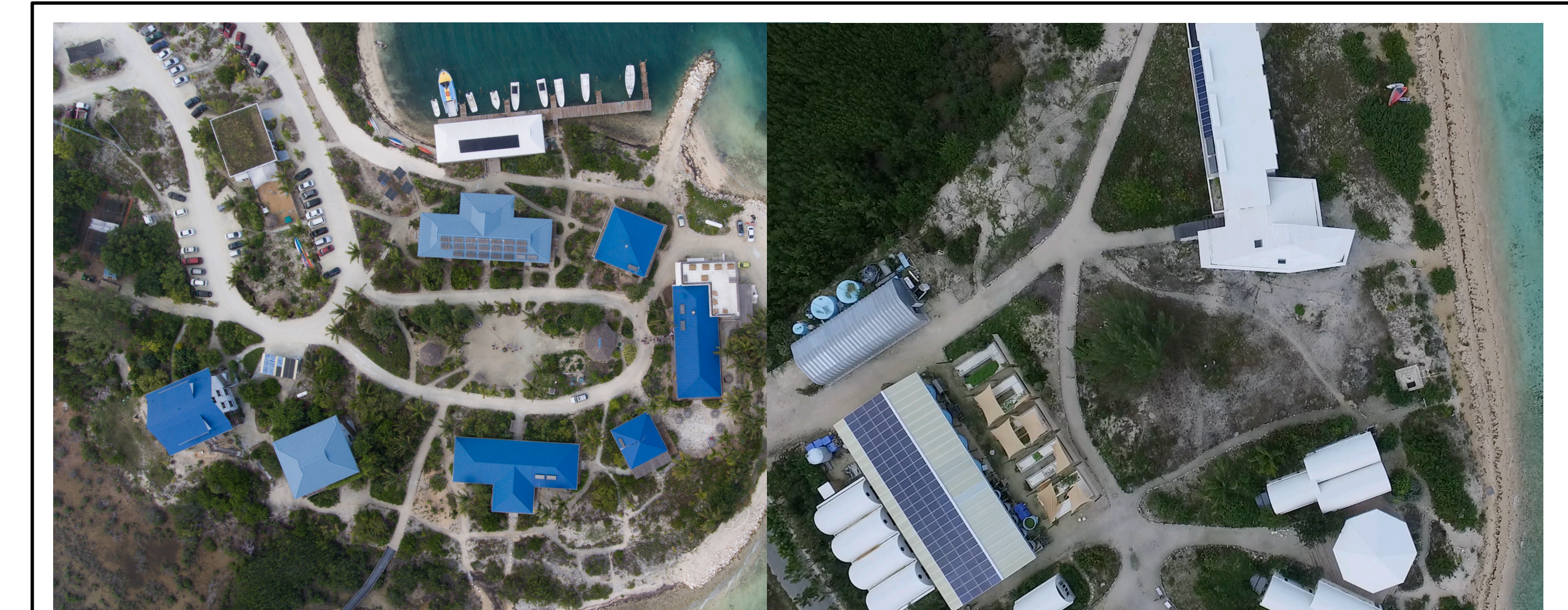
Figure 5: Existing grid-connected solar resources on CEIS campus.
